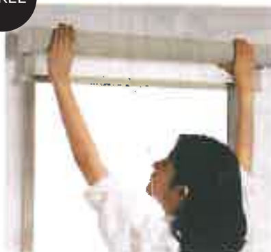
Fit the headbox onto the blind, by sliding the headbox endcaps over both sides of the blind
