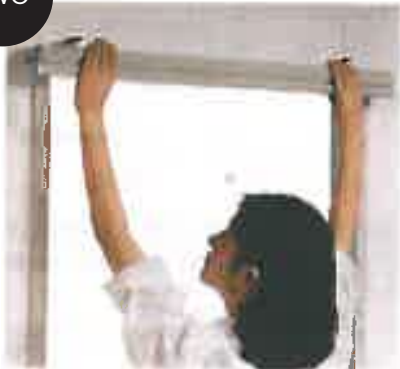
Fit the blind into the brackets
