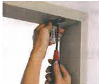
Fix brackets with screws Top Fix [Inside Mount]
