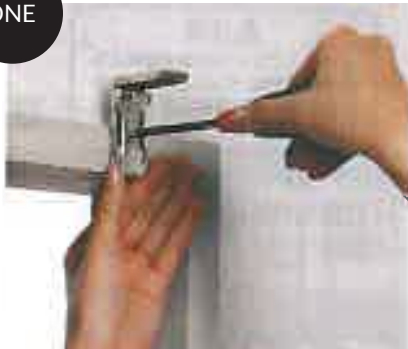
Fix brackets with screws Face Fix [Outside Mount]
